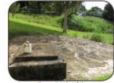
Keep septic tanks sealed.
