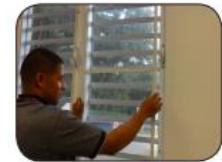
Install or repair window & door screens.
