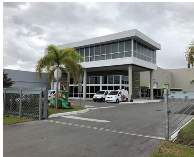
Figure 2-8: Example of Recent Development
