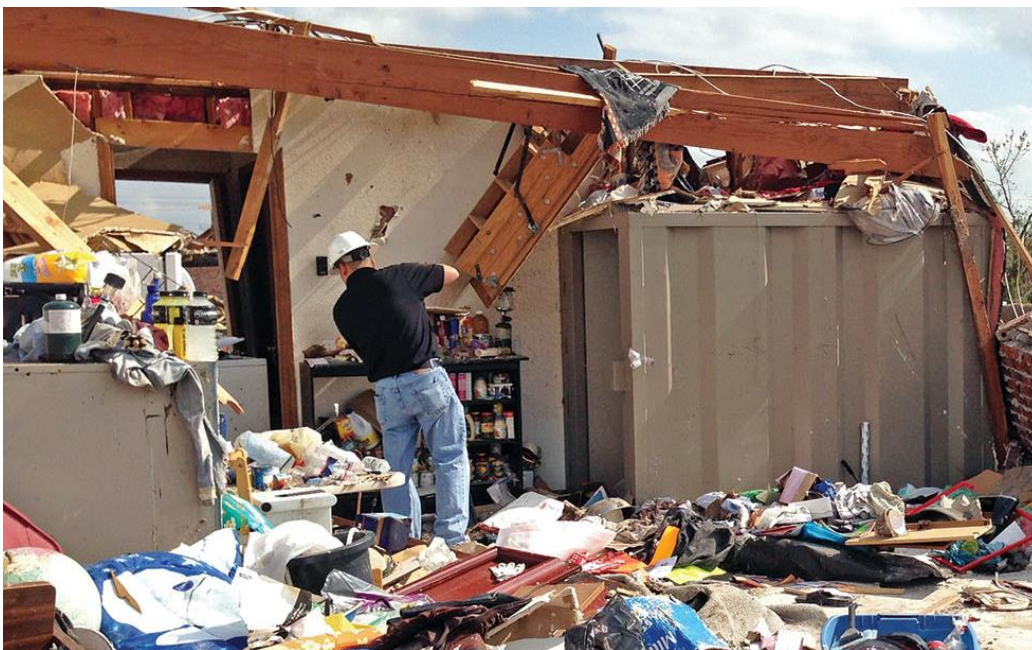
Figure 3. A local building code inspector inspects an above-ground shelter that performed well in a heavily damaged area
