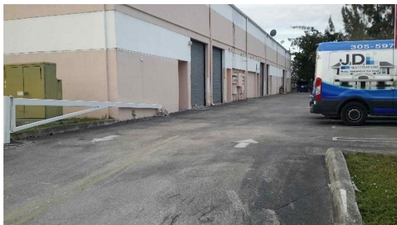
Repetitive Loss Area 12 – Building is elevated above street grade and parking lot
