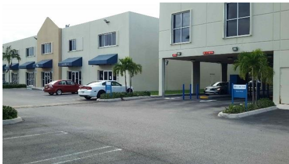
Repetitive Loss Area 17 - Parking lot slopes toward building
