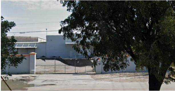
Repetitive Loss Area 8 – Building at below grade; parking lot slopes toward building
