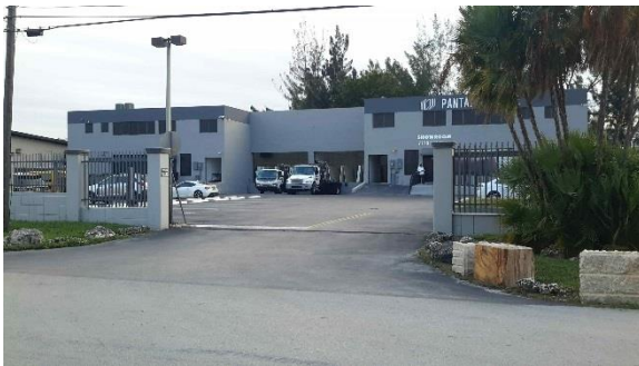
Repetitive Loss Area 10 – Building elevated but inside warehouse is below grade
