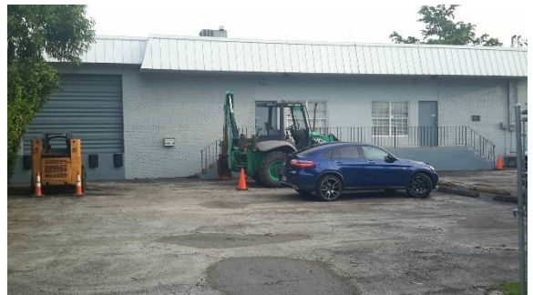
Repetitive Loss Area 2 - Building interior elevated with warehouse/garage area still at grade
