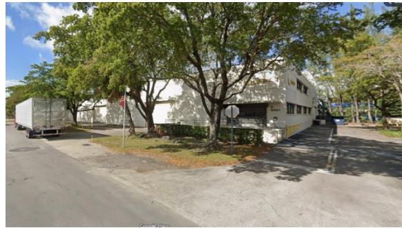
Repetitive Loss Area 16 – Building at grade and parking lot slopes toward building
