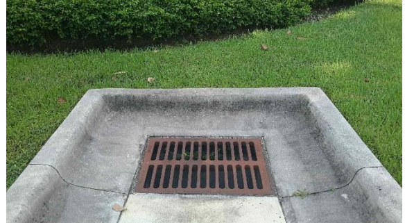
Drainage inlet on corner of block; curb may block entry of water
