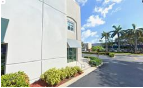
Repetitive Loss Area 14 – First floor offices sit slightly above grade
