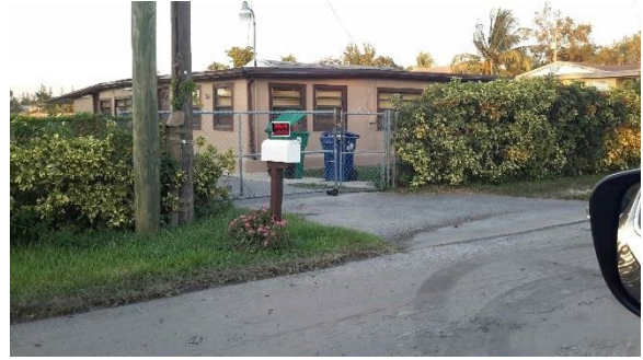
Repetitive Loss Area 21 - House below grade
