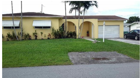
Repetitive Loss Area 18 - House slightly elevated with drainage inlet in front yard
