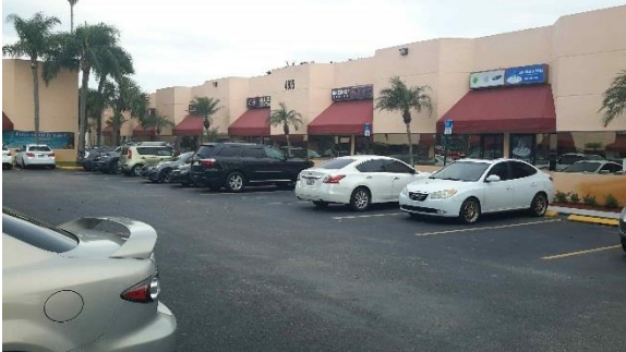
Repetitive Loss Area 7 – Building at grade; water could enter easily from parking lot
