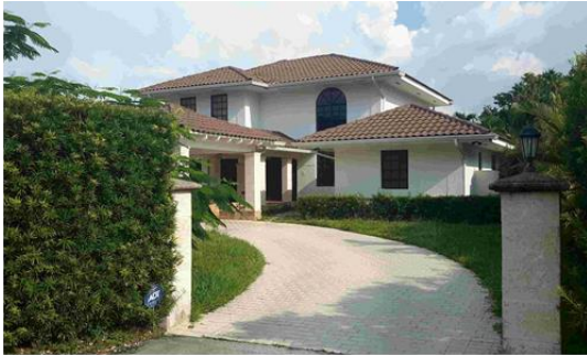
Property elevated slightly above grade
