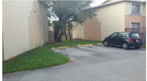
Repetitive Loss Area 7 – Buildings at grade; no guttering
