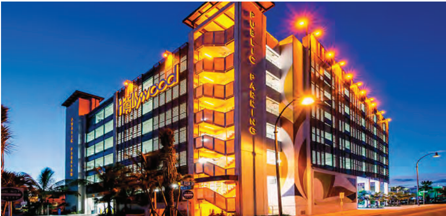
HOLLYWOOD NEBRASKA ST. PARKING GARAGE $13.1 MILLION
