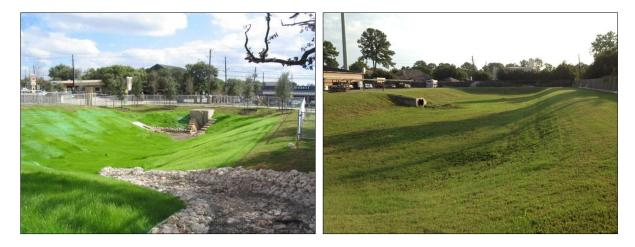
Figure 6-21 – Typical Dry Retention Pond
