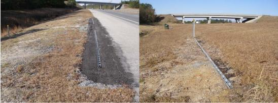
Figure 4. Edge-of-pavement slot drain.
