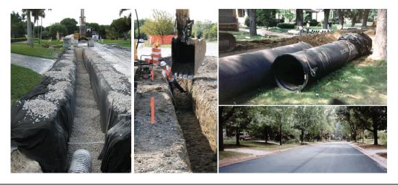
Figure 6-13 – Exfiltration Trench
