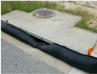
Figure 10-2 - Storm Drain Inlet Protection (b)
