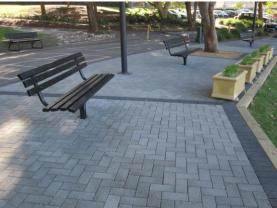
Figure 6-19 - Permeable Pavement in Parking Lot and Park/Walkaway Area
