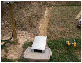
Figure 2. Level spreader, recollection trough, and weir box.
