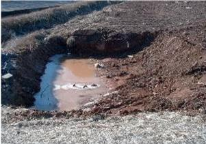
Figure 10-4 – Sediment Trap & Spillway
