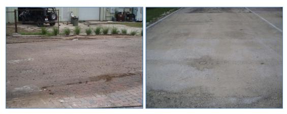
Figure 2 (a) Sandy sediment loaded surfaces (b) Fine limestone dust loaded surfaces
