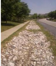
Figure 6-11 – Infiltration Trench
