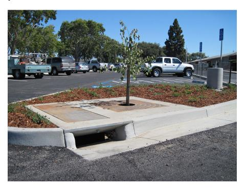
Figure 12 - Newly Installed Urban Green BioFilter
