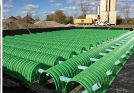
Figure 6-24 – Stormwater Chambers
