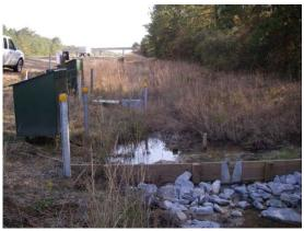
Figure 8. Outlet structure for swales.
