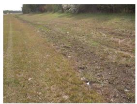
Figure 2 Example of a vegetated swale without wetland characteristics (i.e. standard dry swale).
