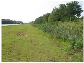
Figure 1. Example of a vegetated swale with wetland characteristics.
