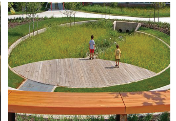
I. Dry Retention Pond
