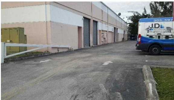
Repetitive Loss Area 15 – Building is elevated above street grade and parking lot
