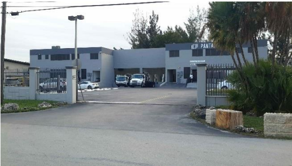
Repetitive Loss Area 13 – Building elevated but inside warehouse is below grade
