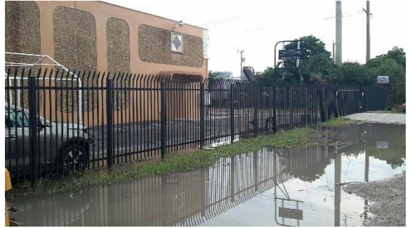
Repetitive Loss Area 7 – Water ponded in parking lot
