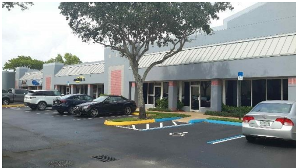
Repetitive Loss Area 25 – Building at grade; parking lot is sloped to catch and drain water
