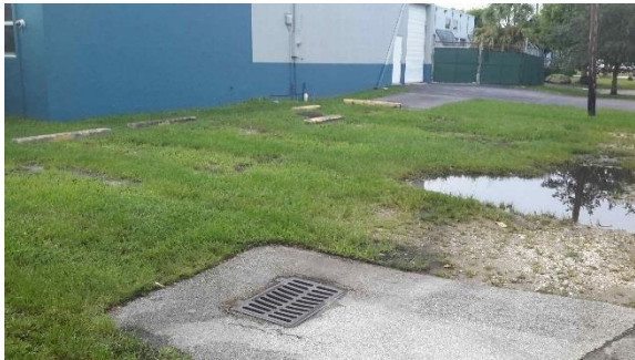
Repetitive Loss Area 8 – Water ponding in lot and not reaching drainage inlet
