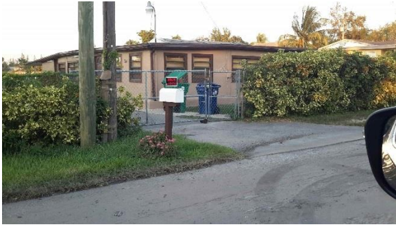
Repetitive Loss Area 17 – House below grade
