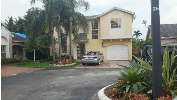
Repetitive Loss Area 1 – Property elevated slightly above grade
