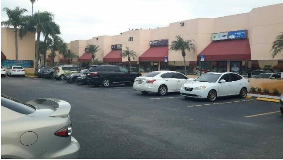
Repetitive Loss Area 10 – Building at grade; water could enter easily from parking lot
