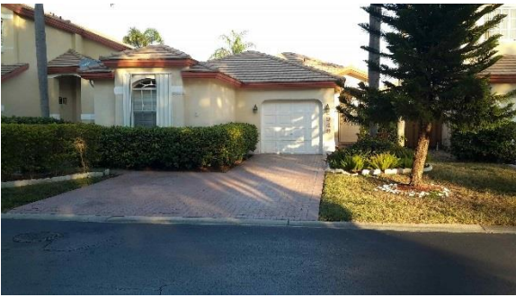
Repetitive Loss Area 16 – House at grade without guttering
