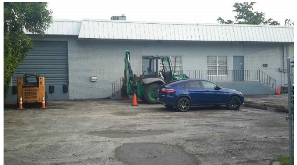
Repetitive Loss Area 9 – Building interior elevated with warehouse/garage area still at grade
