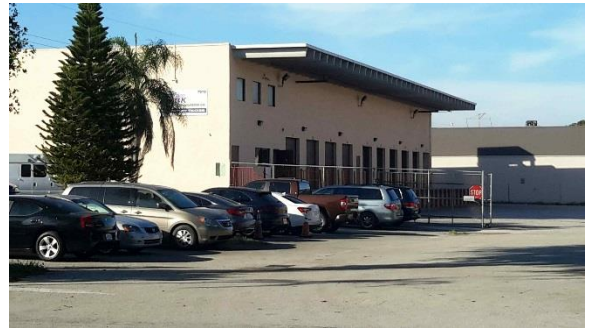
Repetitive Loss Area 14 – Inside of building is elevated
