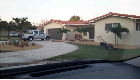
Repetitive Loss Area 18 – Road and driveway slope toward house
