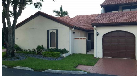
Repetitive Loss Area 4 – House with elevated HVAC and full guttering
