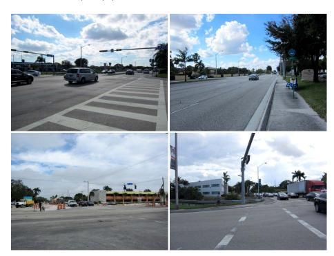
While some of Doral's intersections have clearly marked crosswalks with crossing signals (Top Left), the majority of intersections reviewed in this study were either missing crosswalk striping (Bottom Left), were too far away from transfer points (Upper Right), or were in need of crosswalk striping repainting or missing crossing signals (Bottom Right).
