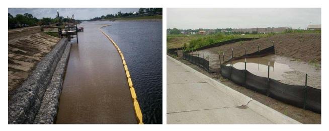
Figure 10-3 – Stacked Turbidity Barrier or Silt Fence (c)
