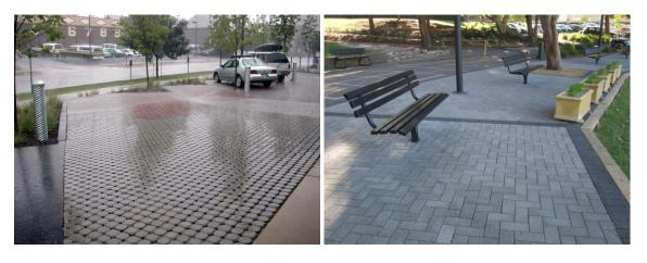
Figure 6-19 – Permeable Pavement in Parking Lot and Park/Walkaway Area
