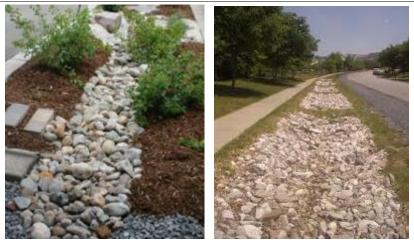
Figure 6-11 – Infiltration Trench
