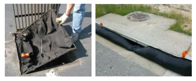
Figure 10-2 – Storm Drain Inlet Protection (b)
