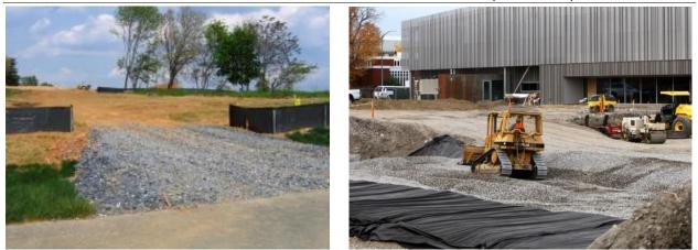
Figure 10-1 – Temporary Gravel Construction Entrance & Exit (a)
