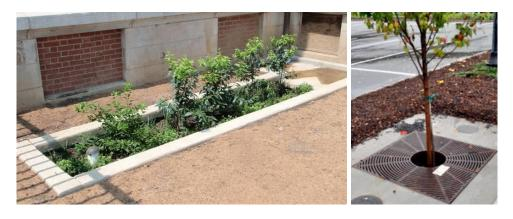
Figure 6-4 – Infiltration Planter and Tree Box
