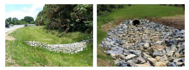
Figure 10-6 – Stone Check Dams in Swale and Stone Outlet Trap
