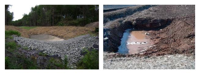
Figure 10-4 – Sediment Trap & Spillway
