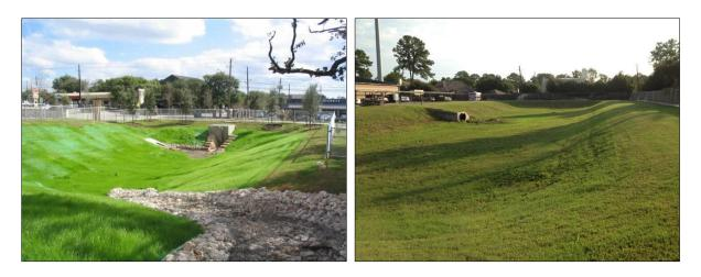
Figure 6-21 – Typical Dry Retention Pond
