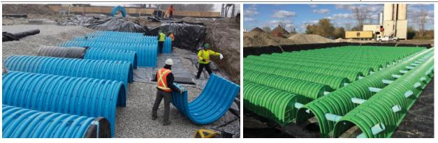
Figure 6-24 – Stormwater Chambers
