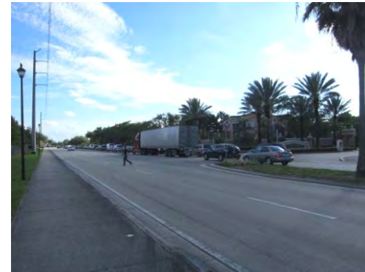
Pedestrian jaywalking on NW 107 th Avenue. Observations of jaywalking can be an indication of “desire lines” on roadways. Such areas should be studied further for possibility of a mid-block crossing.
