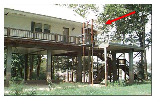
Figure 8-6. Elevator provides access to elevated structure
