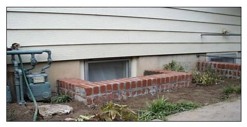
Figure 7-4. Low wall construction
