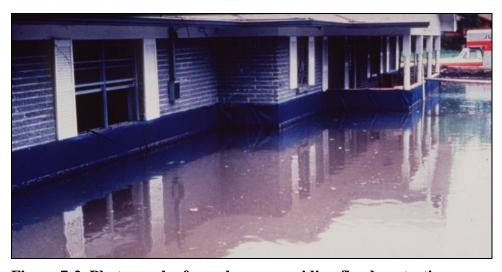
Figure 7-2. Photograph of membrane providing flood protection
