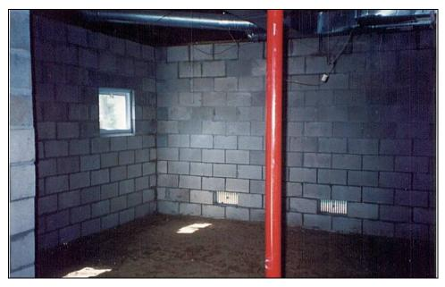
Figure 8-4. New foundation with vents
