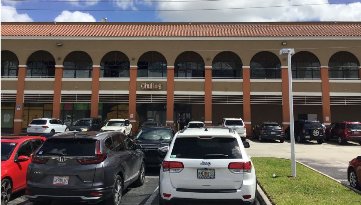
Figure 5-14: Commercial building 79th Ave in the Area of Influence
