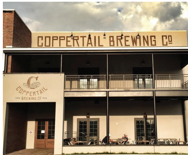
Figure 2-3: Coppertail Brewing, Tampa, FL is an example of an adaptive reuse brewery development. Source: The Trot Line: www.setthetrotline.com/2015/04/14/start-your-tampa-brewery-tour-at-coppertail-brewing-co/
