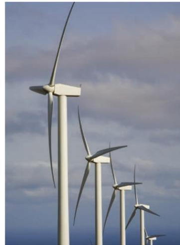
Height is an important consideration when using wind power. The wind increases with additional height above the ground. The wind power available at 100 feet is typically twice the power available at 30 feet.
