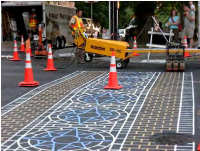
Painted/textured crosswalks can be achieved through the application of thermoplastic striping, and applied to raised crosswalks as well.
