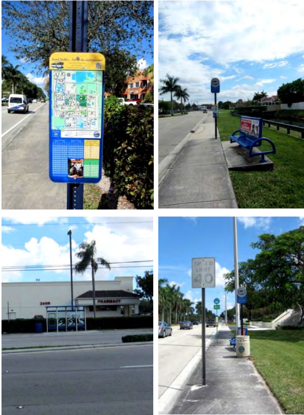
Bus stop amenities utilized within Doral include well designed trolley maps for wayfinding (Top Left), distinct bus signs and benches for transit riders waiting for the Trolley (Top Right), bus shelters at some stops, providing shade and seating and trash cans (Bottom Left). Some stops serve as transfer points between the Trolley and MDT buses, with shared amenities such as seating and waste disposal (Bottom Right).
