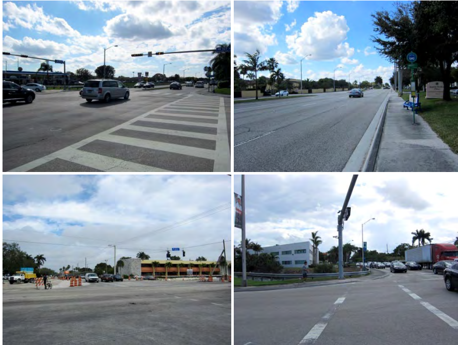
While some of Doral’s intersections have clearly marked crosswalks with crossing signals (Top Left), the majority of intersections reviewed in this study were either missing crosswalk striping (Bottom Left), were too far away from transfer points (Upper Right), or were in need of crosswalk striping repainting or missing crossing signals (Bottom Right).
