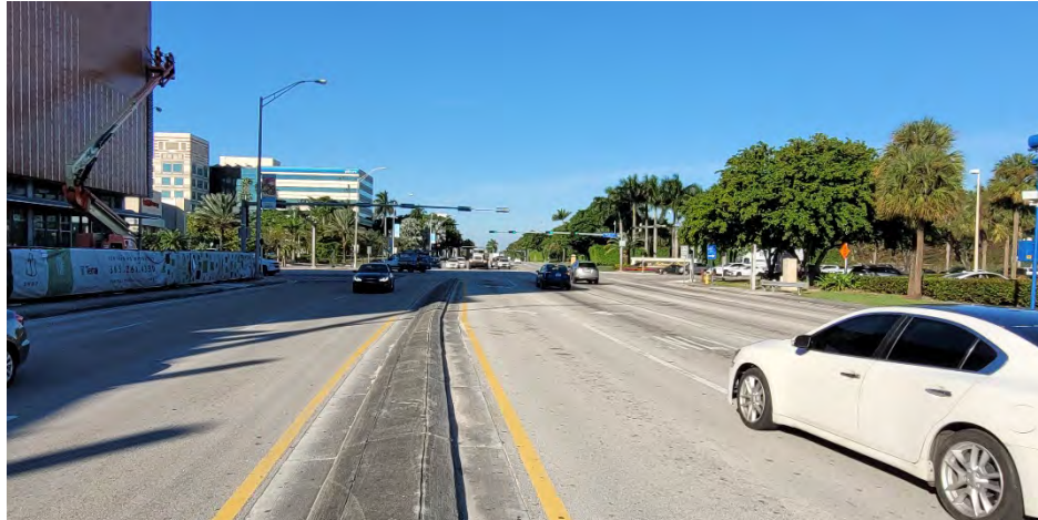
Photo 21: Westbound view to the NW 87th Ave signal
