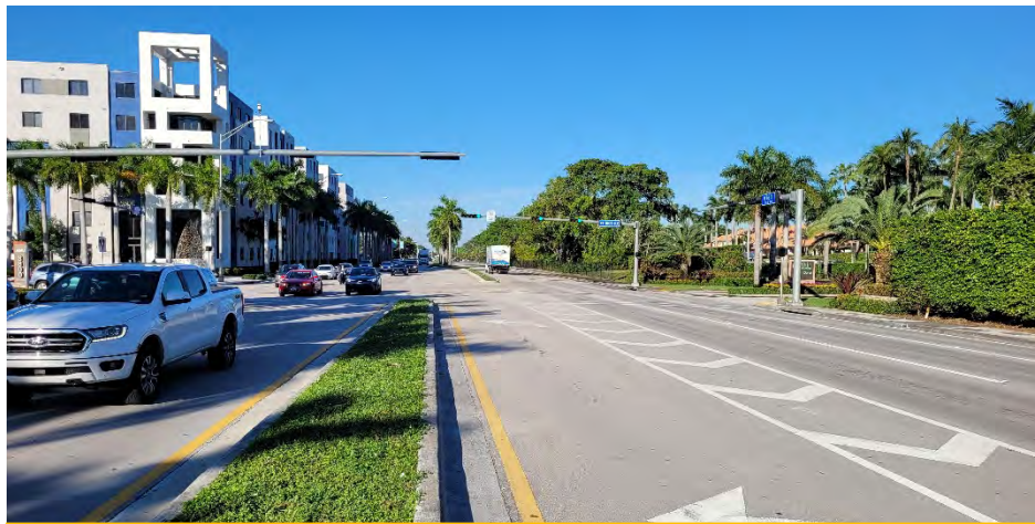
Photo 15: Westbound view to the NW 8800 Block signal
