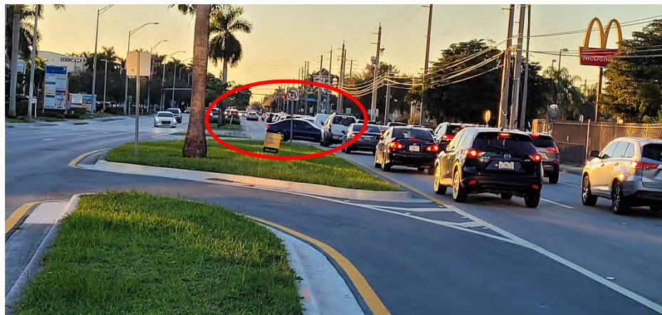
Photo 47: View of eastbound vehicle making a U-turn among stopped westbound vehicles at Median Opening #4
