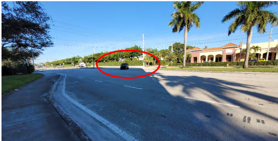
Photo 24: Southbound left-turning at Median Opening #16
