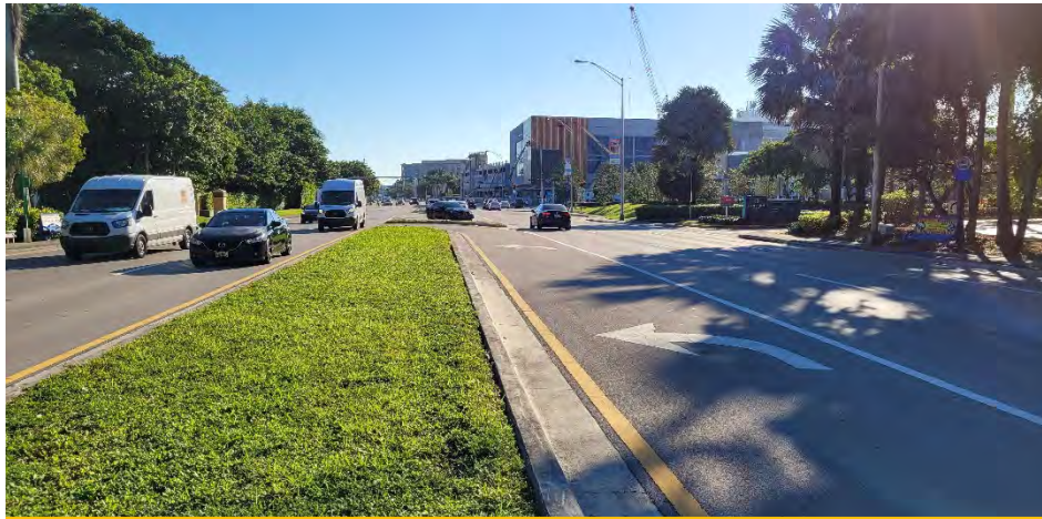
Photo 17: View of eastbound approach to Median Opening #13
