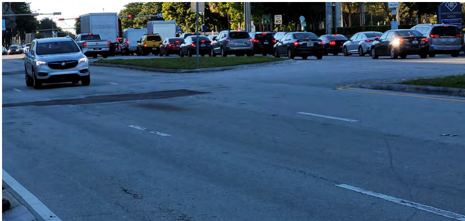
Photo 52: View of westbound approach vehicles to the NW 87th Ave signal
