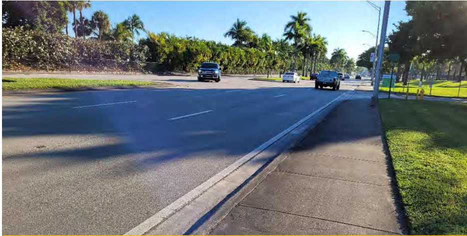
Photo 12: Typical View of traffic conditions at MO#s 7 through 12
