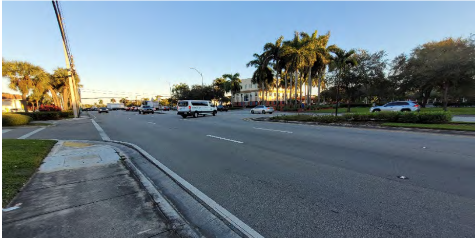
Photo 38: Southbound vehicle turning left from Median Opening #1
