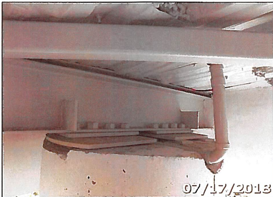
PHOTO 08: West Bearing Overview
