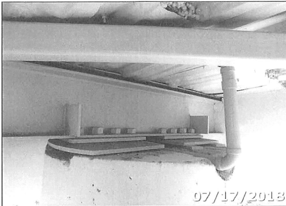
PHOTO 08: West Bearing Overview
