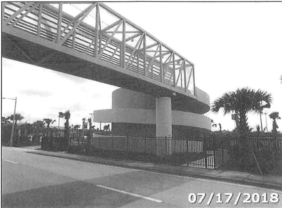
PHOTO 06: East Column and Circular Ramp Overview
