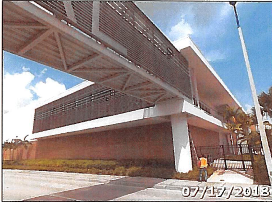
PHOTO 05: West Column Overview
