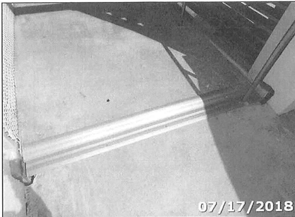
PHOTO 04: Typical Expansion Joint
