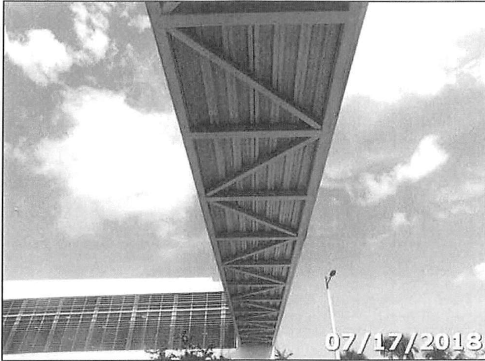
PHOTO 07: Deck Underside Overview
