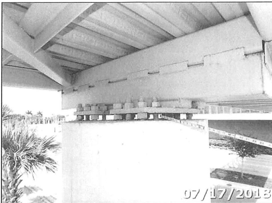
PHOTO 09: East Bearing Overview
