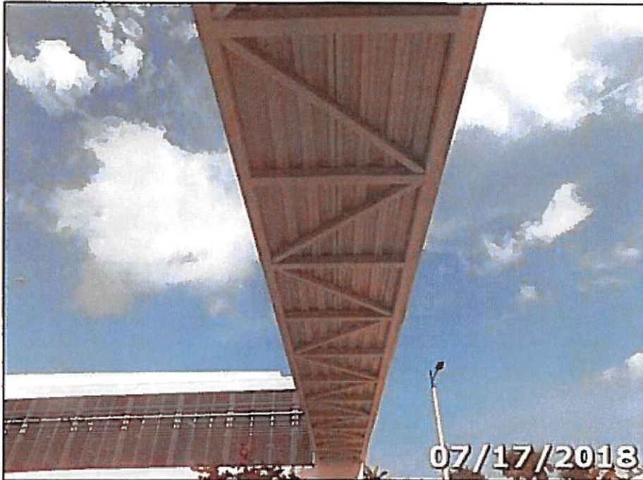
PHOTO 07: Deck Underside Overview
