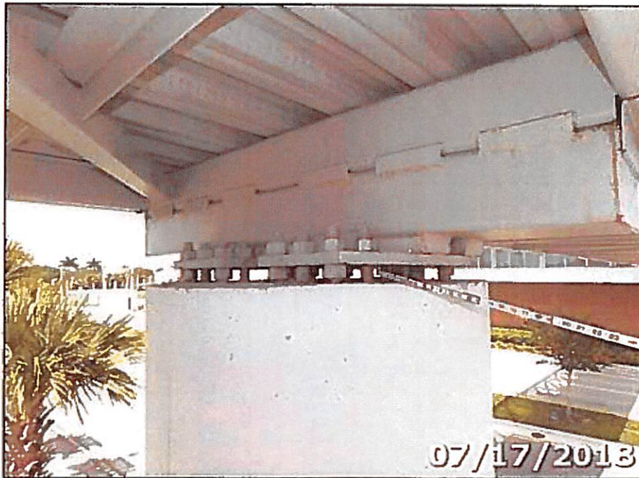
PHOTO 09: East Bearing Overview
