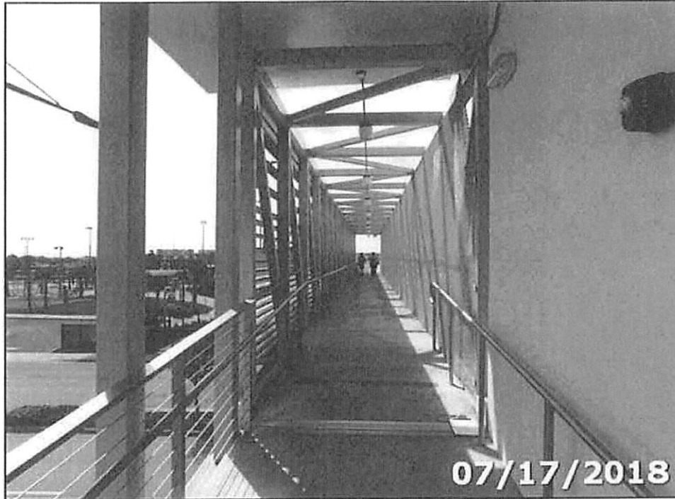
PHOTO 03: Deck Overview (West entrance Looking East)
