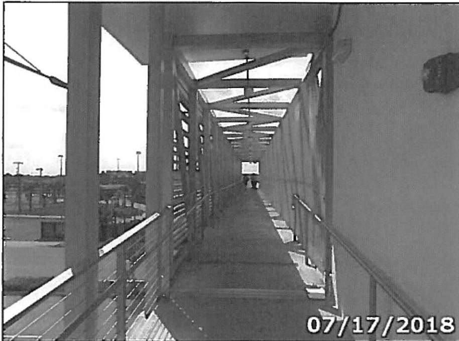
PHOTO 03: Deck Overview (West entrance Looking East)
