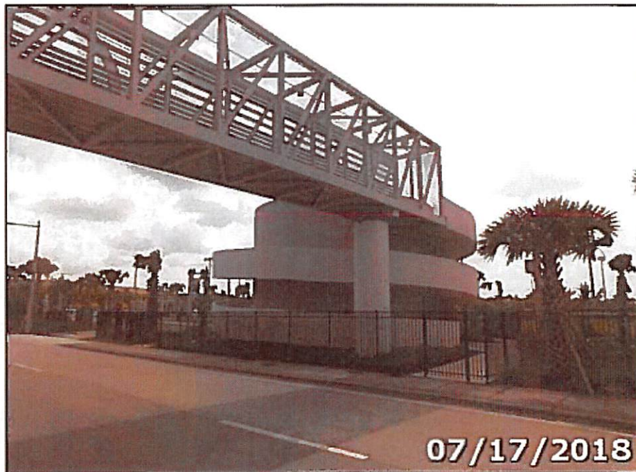
PHOTO 06: East Column and Circular Ramp Overview
