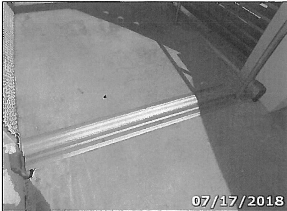
PHOTO 04: Typical Expansion Joint
