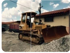
CAT D3G Dozer
