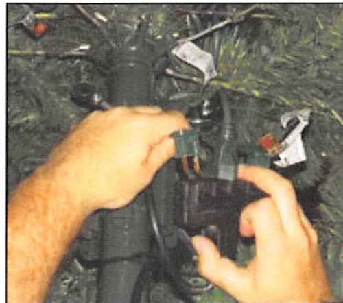
Electrical Harness with Extension Cord and Topper Light Plug Attached
