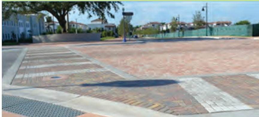
Decorative Pavers (Roadway)
