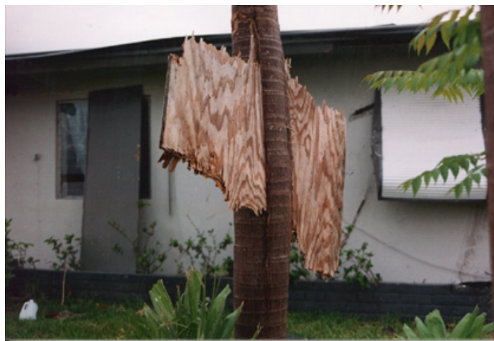
Damage showing impact of Hurricane speed winds
