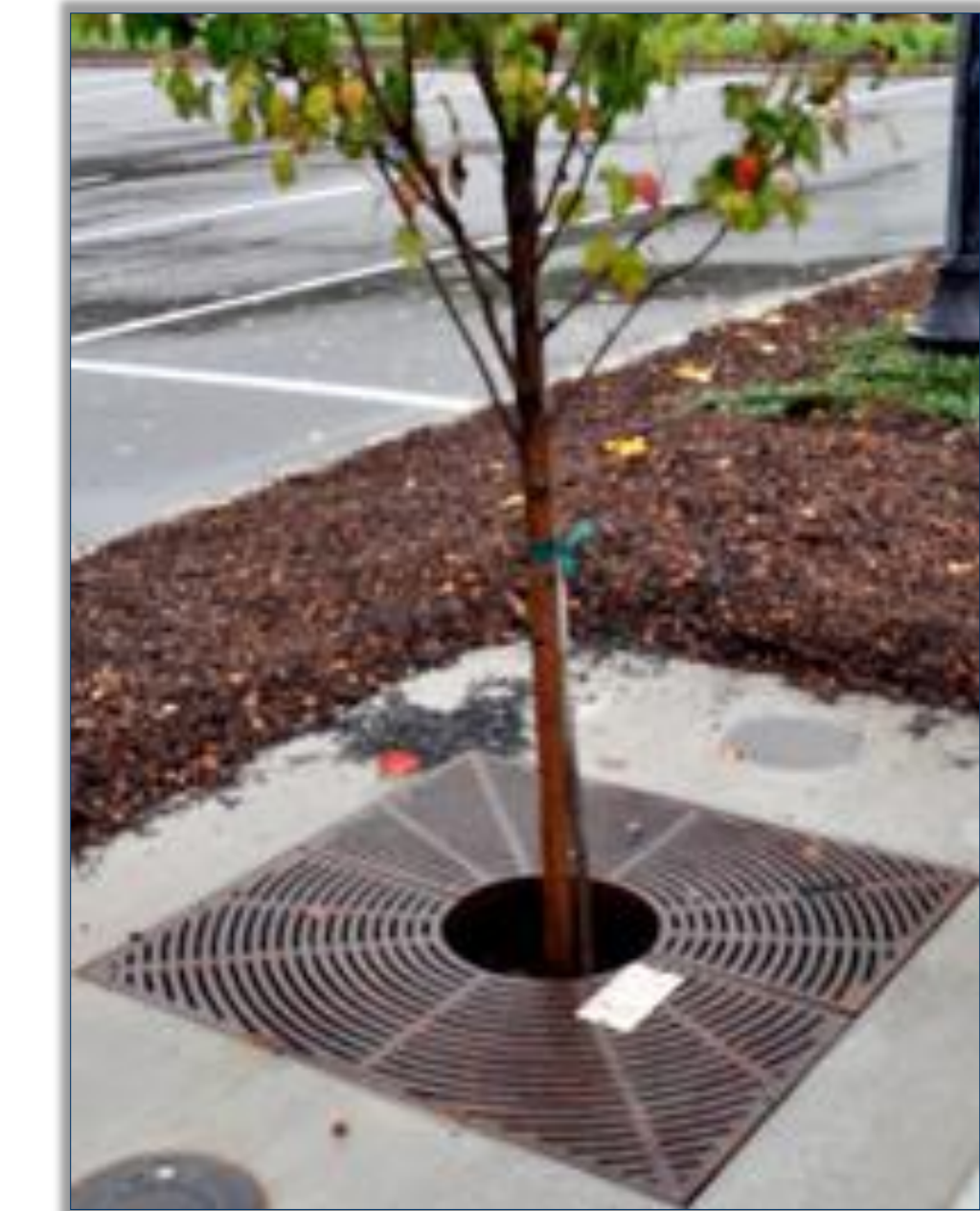
Tree Box Filters or Infiltration Planters
