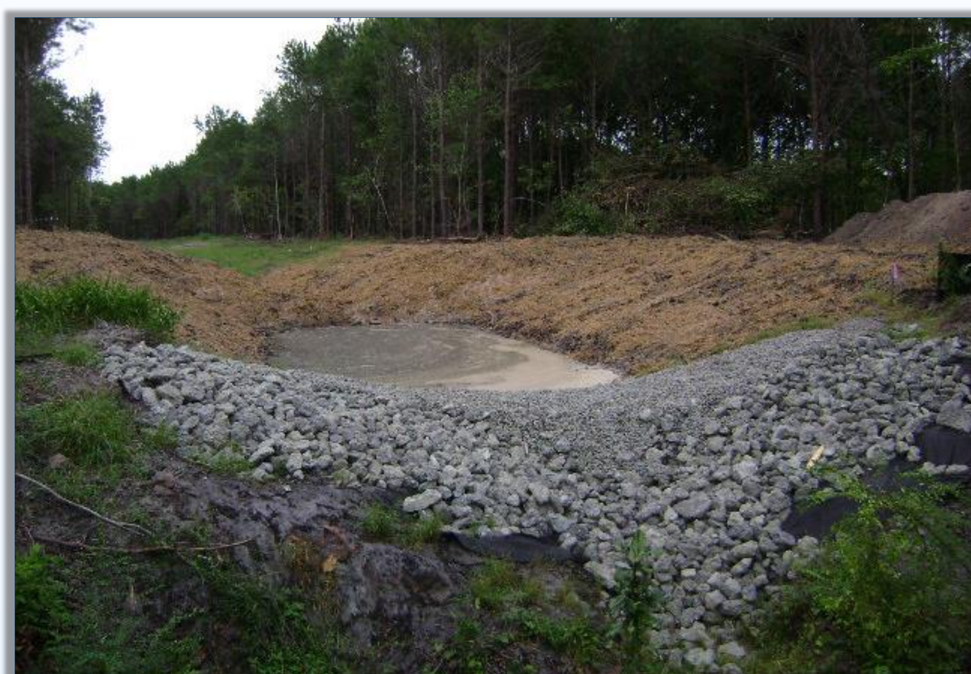
Runoff Trap & Spillway
