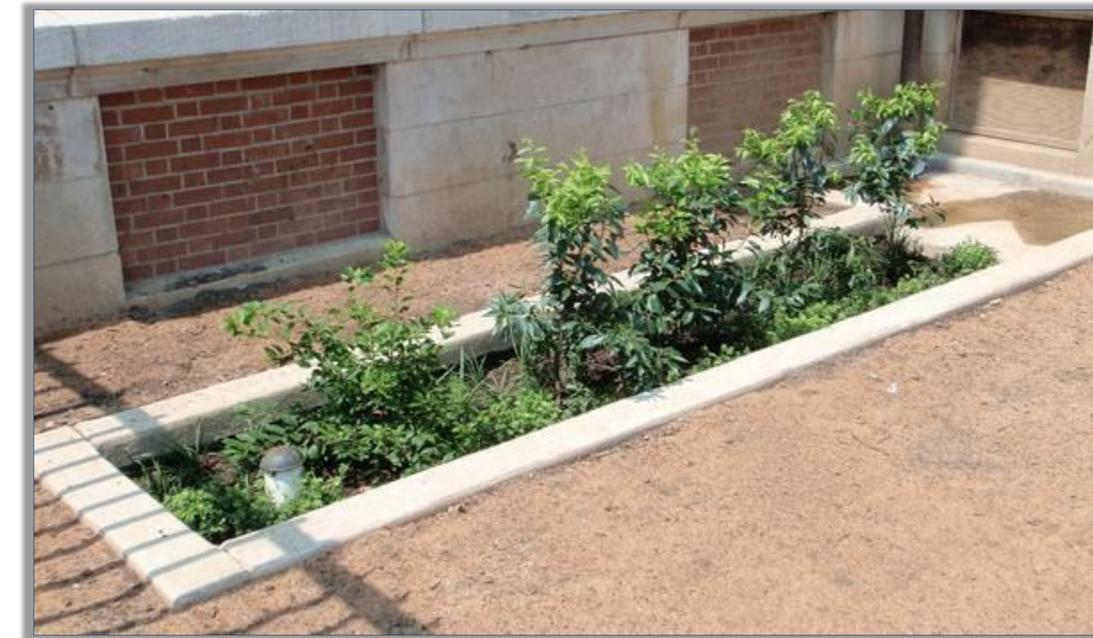
Tree Box Filters or Infiltration Planters
