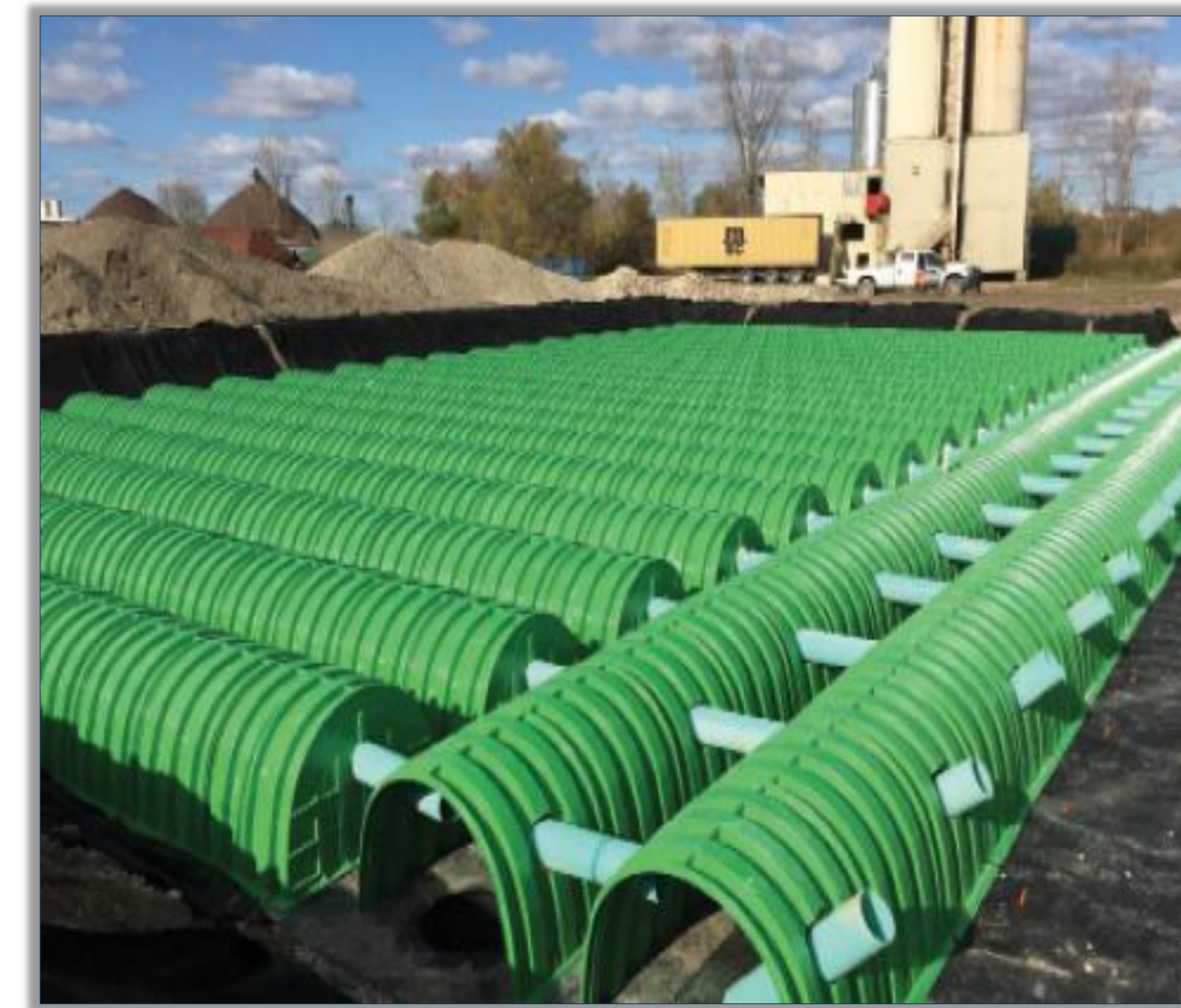
Parking Stormwater Chambers
