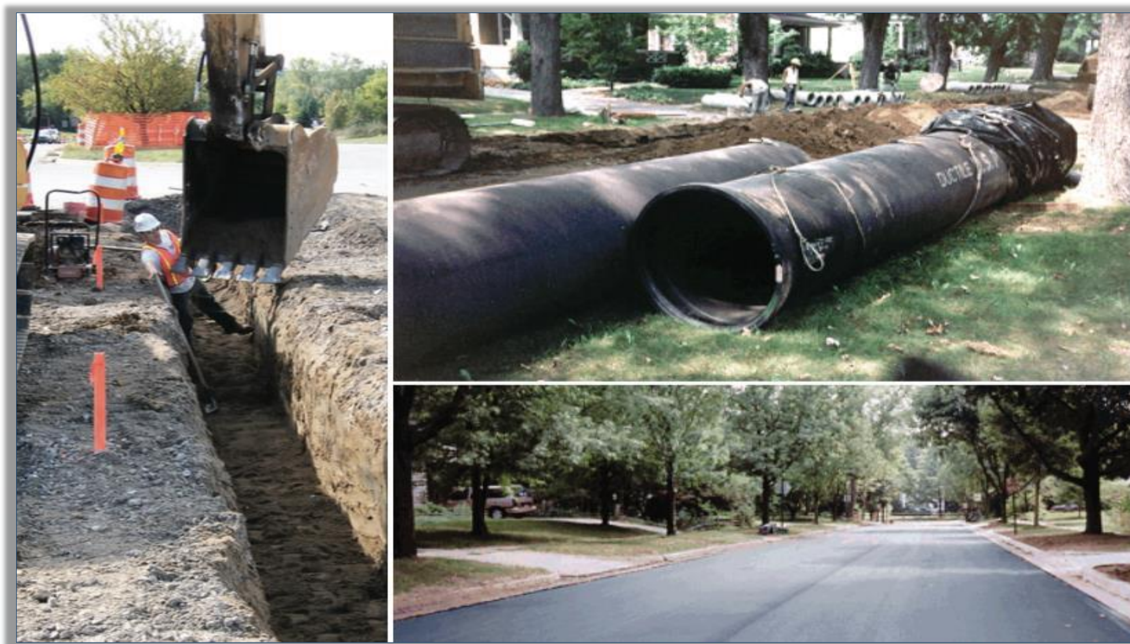
Exfiltration Trench or French Drain
