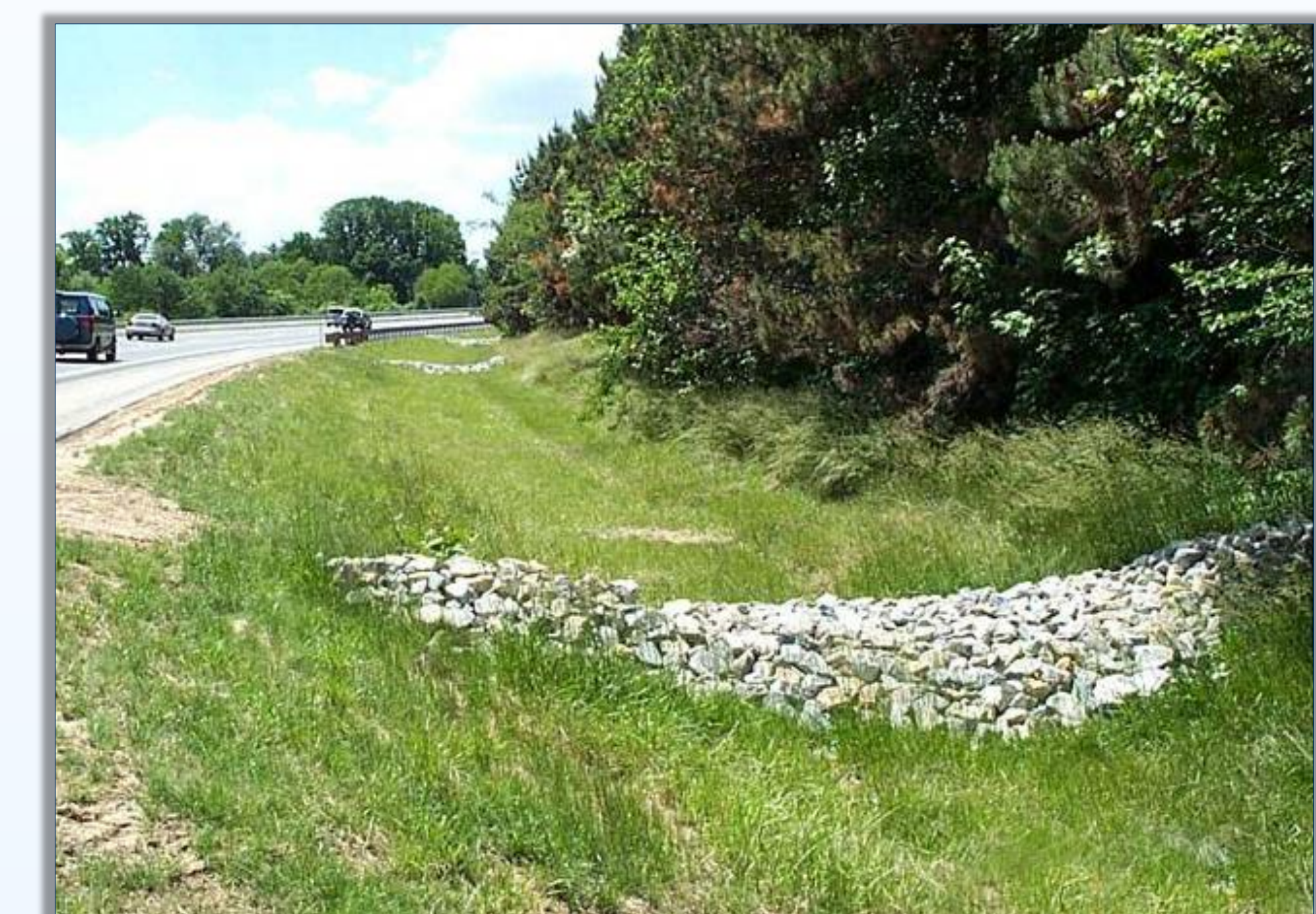
Stone Check Dam
