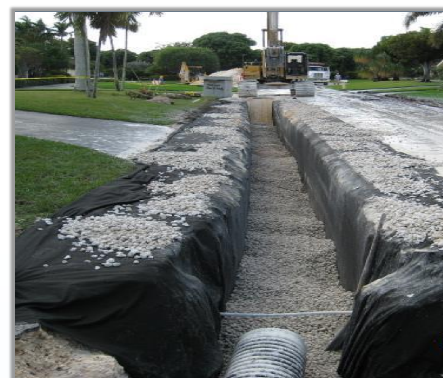
Exfiltration Trench or French Drain
