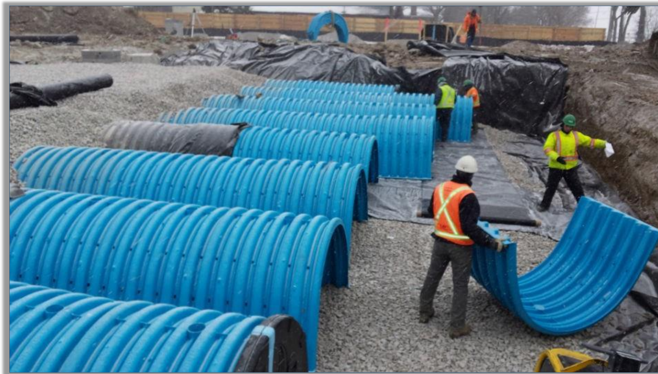
Parking Stormwater Chambers
