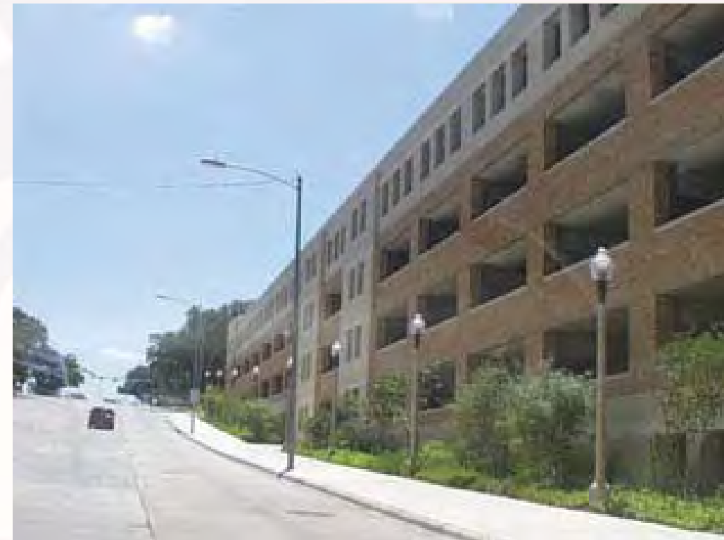
Garage parking use immediately abutting the sidewalk, as shown above, creates a void along the activity zones of sidewalks and are highly discouraged by this master plan.
