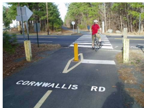
Shared Use Path / Roadway Crossing
