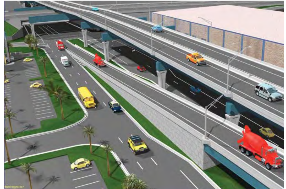
Looking northwest at Viaduct
